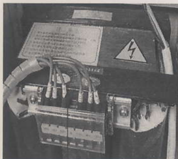
Transformer 3P 380V/3P 220V
